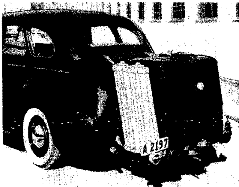
Figure 129. Folding (i.e., Back-swinging) Charcoal Gas Generator for a Passenger Car.
