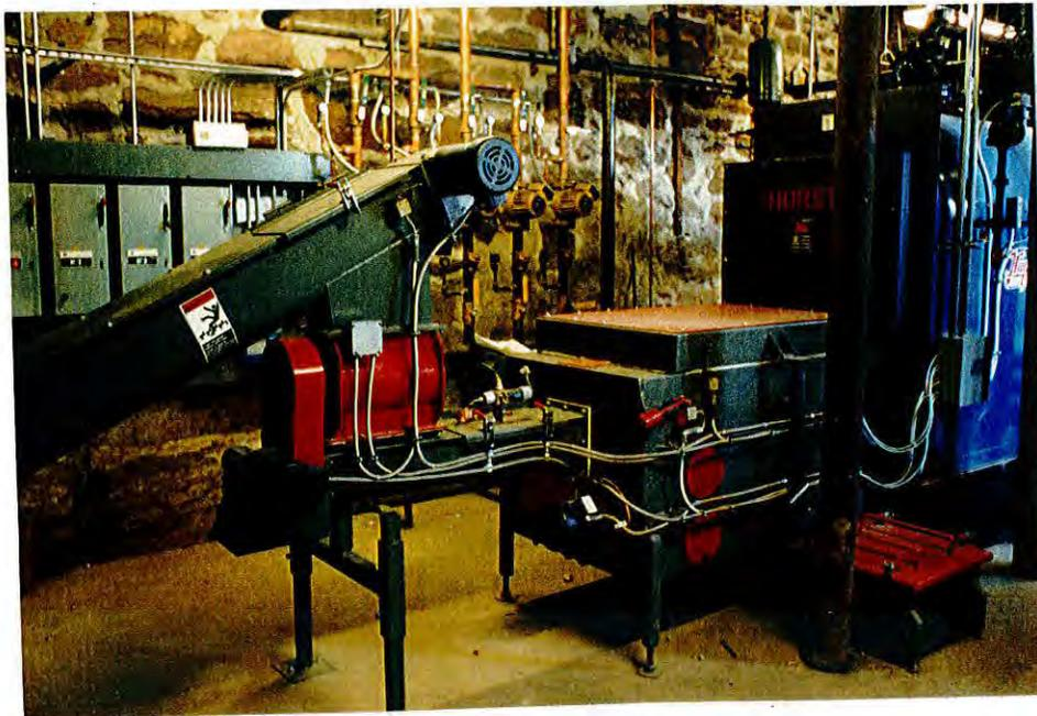
**Figure 1 - A Chiptec C-2 gasifier (2M Btu/hr) powering a Hurst SI-50 Boiler**
